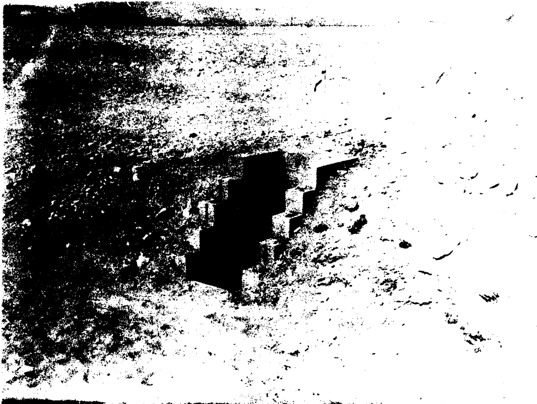
Fig. 10—Entrance to block-wall basement exit before blast.
